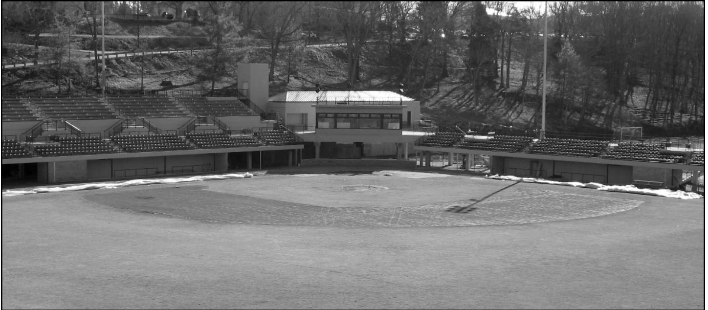
After over a year of construction, the Keydets will open Gray-Minor Stadium this February.
