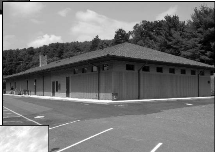
At right, the Patchin Field Locker Room Complex, which houses locker rooms for the Keydets' baseball, lacrosse, women's soccer and men's soccer teams, as well as a visiting locker room, an officials' locker room, as well as an athletic training facility.
